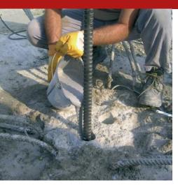
An anti-shrinkage, pourable, self-levelling, super-adhesive micro-mortar, based on highstrength cements, super-pozzolanic fillers, polymeric stabilisers and anti-shrinkage agents. Aggregates with a maximum size of 0.35 mm. Ideal for consolidating and reinforcing injections on concrete, masonry and cracked/damaged rock. Anchors and fastens steel bars, pins, brackets and so on, to concrete, masonry and rock.
