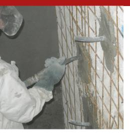
Super-fluid, injectable, cementitious grout with very high flowability and stability, moderately expansive in the plastic phase, for fixings, anchors, wall consolidation, fillings, filling of post-tension sheaths, etc., based on high-strength cements, specific additives, fillers superpozzolanic reagents. Maximum particle size 0.06 mm.
