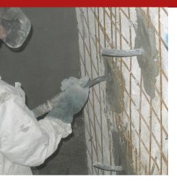
Super-fluid, injectable, cementitious grout with very high flowability and stability, moderately expansive in the plastic phase, for fixings, anchors, wall consolidation, fillings, filling of post-tension sheaths, etc., based on high-strength cements, specific additives, fillers superpozzolanic reagents. Maximum particle size 0.06 mm.
