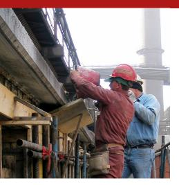
Grout 6 is a high-performance, self-levelling pourable mortar that is fibre-reinforced with Readymesh PM-060 microfibres, with high durability even in aggressive environments, great adhesion on concrete and steel and compensated shrinkage. Aggregates with a maximum size of 6 mm. It is ideal for restorations, reinforcements and seismic adjustments for medium-to-high thicknesses (4–15 cm), on structures in reinforced concrete and masonry.
