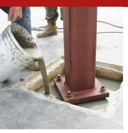
Grout 2 is a high-performance, self-levelling pourable mortar that is fibre-reinforced with Readymesh PM-060 microfibres, with high durability even in aggressive environments, great adhesion on concrete and steel and compensated shrinkage. Aggregates with a maximum size of 2 mm. Ideal for anchoring machinery with subplate casting, anchoring seismic isolators and embedding bars, for repairs and reinforcements that are quite thin (2–6 cm) on reinforced concrete and masonry structures.
