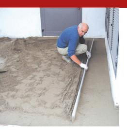
Ready-mixed, composite , reinforced fibre conglomerate, for construction, with the sole addition of mix water, of paving slabs with a thickness between 40 and 60 mm, laid with the consistency of "damp earth".
