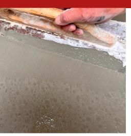
Floor Level is a self-levelling modified-polymer cement mortar with fibre-reinforcement, offering accelerated grip and fast hardening. Applied prior to laying the flooring, it is perfect for levelling at thickness ranging from 3 mm to 20 mm so as to adapt to any type of covering.
