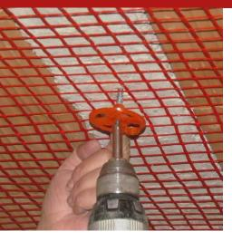
Nylon fastening flange (58 mm in diameter and 40 mm in length) with self-tapping screw in corrosion-resistant galvanised steel (30 mm) for connecting ARMAGLASS STRUCTURA mesh in anti-detachment RINFOR SYSTEM 1 and 2.
