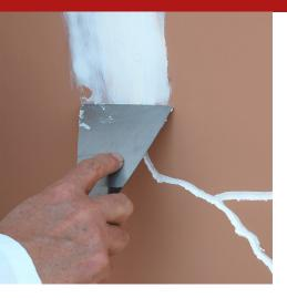
Adhesive filler, white in colour, for grouting and filling cracks and fissures and small imperfections on plasters and external walls, also in combination with Sanaxil Filler.
