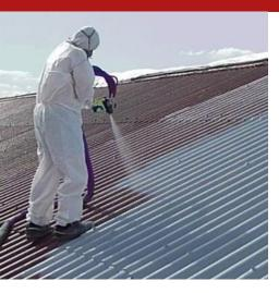
One-component coating based on acrylic resins in aqueous dispersion for permanent encapsulation of type A (visible outside), B (visible inside) and C (not visible, before confinement) of asbestos sheets , certified in accordance with the DM August 20, 1999. Elastocap-ABC is characterized by high flexibility, resistance to yellowing, adhesion and creates a waterproof and crack-resistant membrane.
