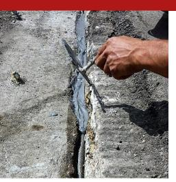
Epoxy-polyurethane two-component elastoplastic and thixotropic sealant, for joints subject to traffic, where Shore A Hardness Scale = 65. The elongation-at-break is 70%. To be applied with a trowel or extruded into the suitably-taped sections of the joint (to protect adjacent surfaces). Resistant to contact with hydrocarbons (gasoline and diesel fuel).
