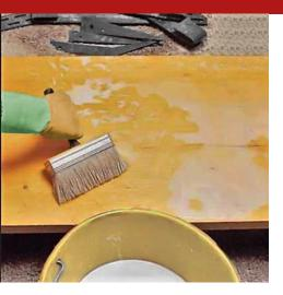
Anti-adhesive release agent, emulsifiable in water, based on aromatic alkylates and specific agents, for easy removal of wooden formworks during dismantling. To be applied by spraying or roller to formworks dry and free of any soiling.
