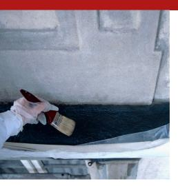
Transparent penetrating consolidator, for natural stones, ornamental stone elements, mineral plasters and in general for the restoration of cultural heritage. It consists of ethyl esters of silicic acid in solvent, hardening by reaction with atmospheric humidity. It is applied by spraying at low pressure, until the treated surfaces are rejected, in order to guarantee an extremely deep consolidation.
