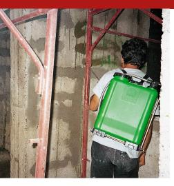
Reactive, colourless mineral solution for preliminarily re-alkalising and reinforcing concrete surfaces to be restored. It is an inorganic, mineral compound chemical affine with concretes. It reacts with alkali hydrates alkaline and with water, present in the porosity of concretes, mortars and plasters, forming stable silicate gels, which hermetically and lastingly seal the capillary lattice.
