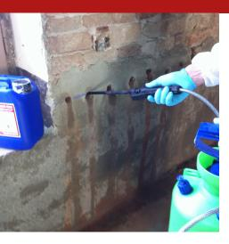
Aqueous, water repellent microemulsion based on low molecular weight silane monomers, free from polluting solvents and reaction by-products, characterised by very high penetration and considerable reinforcing, protective effectiveness. It does not involve alterations in colour, appearance and breathability of the masonry structure. Suitable for forming horizontal chemical barriers against rising damp, free from awkward reaction waiting times.
