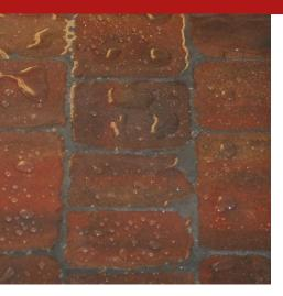
Consilex EM Drop is a VOC-free aqueous silane emulsion used to make absorbent building materials water-repellent and confer a high pearl effect. A water-repellent, colourless, non-filming impregnator to protect plasters, cement systems, and so on, without altering the treated surfaces.
