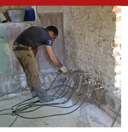
Solution of special modified silicone resins, dispersed in water, hydrophilic in the application phase, water-repellent and water-repellent after reaction with atmospheric carbon dioxide, for the preparation of water-repellent solutions for the creation of chemical barriers against capillary rising in masonry.
