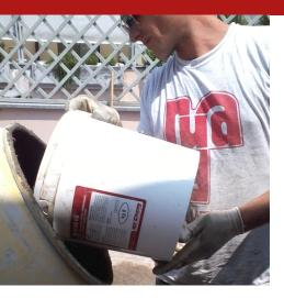
Adhesive multifunctional binding latex, in clear coloured rosy viscous solution, based on a special elastomer in aqueous dispersion, coalescence promoters, de-aerating agents and fillers with superpozzolanic reactivity. Bond HG is a reactive type multifunctional, flexibilising and waterproofing compound, for preparing adhesive grout, waterproofing coatings, and to improve mortar, plaster, grout and concrete adhesion, adherence, deformability, waterproofness and performance.
