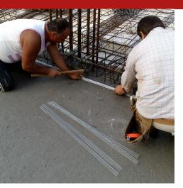
Trapezoid preshaped steel square mesh cage open only on one side, to be used to encourage correct positioning of the Clayseal 25.20 sodium bentonite waterstops, and to prevent the displacement from the seat provided, especially in complex situations or on surfaces which are not perfectly prepared. Once the joint is inserted, Bentonet will have to be fixed to the concrete support using steel nails and washers every 20-25 cm.
