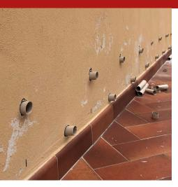
1 metre long stiff paper tube, supplied with 6 plastic closure caps, specific for water repellent resin injections for the construction of slow radial diffusion chemical barriers at the base of the walls, against capillary rising damp, in the brick, tufas, stone, and mixed masonry of various thickness.
