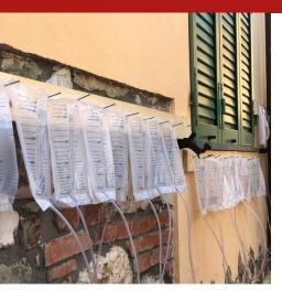
Graduated polyethylene bag, to be fixed by nailing to a suitable wooden or masonry stand, necessary for the chemical barriers against the capillary rising damp with the slow diffusion method.
