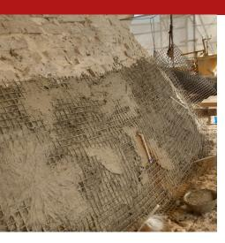
The Armarock B50 basalt mesh is a material with a leno structure, formed by elastic ribs of high-strength basalt threads, fixed in the nodes with a stitching thread, with the formation of square cells, the size of which is ideal for use with FRCM mortars. The mesh is treated with special compounds to improve alkali resistance properties and increase its stability. Balanced biaxial mesh in alkali-resistant basalt fibre, specific for strengthening and repairing structural elements.
