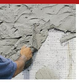
Anti-cracking reinforcement mesh, made of alkali resistant fibreglass yarn, for the best distribution of tensions and to avoid shrinkage cracks caused by changes in temperature, due to lack of planar homogeneity etc. They are available in 3 different types: the  $60~g/m^2$  version, with a 2.7~x~2.7~m square mesh, perfect for reinforced micro-screeds. The standard roll is 1~m in height by 100~m in length.
