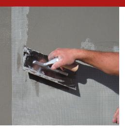
Anti-cracking reinforcement mesh, based on alkaline-resistant fibreglass fibres for better distribution of tension and to prevent cracks from shrinkage, deriving from temperature variations, planar inhomogeneities, etcetera. With a weight of 160 g/m2 and a  $4.5 \times 4.5 \text{ mm}$  square mesh, Armaglass 160 is the ideal fibreglass mesh for creating reinforced skim coats.
